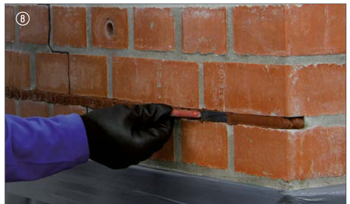
8 DESOI Spiralanker glattstreichen | Flatten out the DESOI Spiral Anchor Mortar
