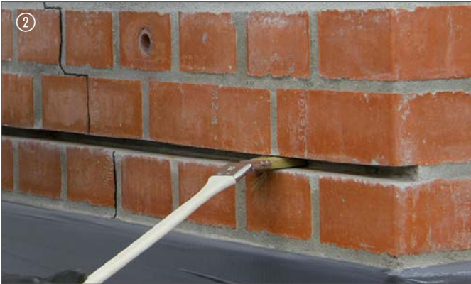
2 Fuge reinigen | Clean the joint/slot
